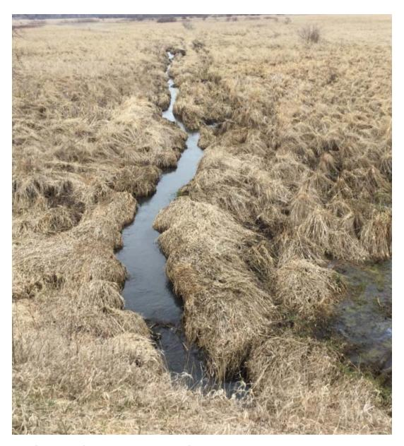
$Photo from \ the \ end \ of \ the \ ditch \ in \ the \ general \ area \ of \ Norway \ Rd \ showing \ narrowing \ and \ alignment \ issues$
